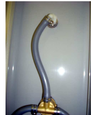
Above flexi pipe leading to overhead shower. Tighten all clips and fixings. Remember to repeat operation to the hand shower connections
