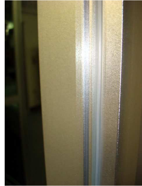
Above shows glass in channel neatly pressed fully in place.
