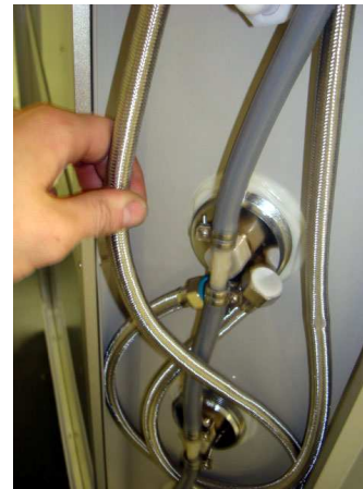
Massage jets tighten white nuts or apply sealer
