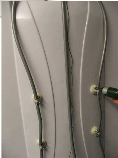
Tighten all hose clips
