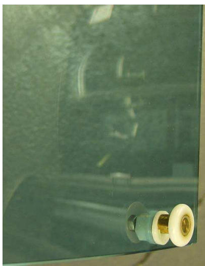
Wheels fit as picture note the cam to adjust
